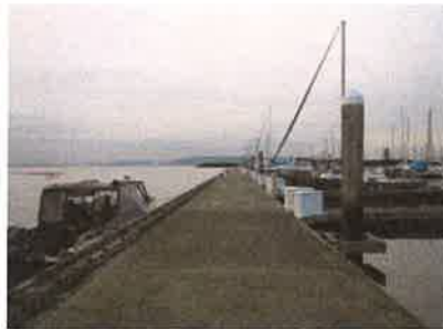
Example of a concrete pontoon floating breakwater.
