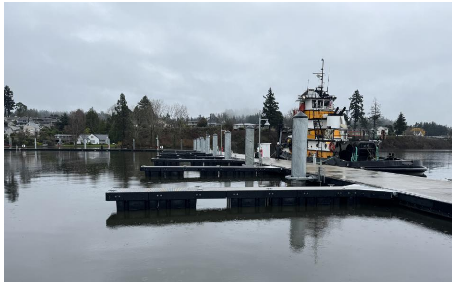
30-ft and 50-ft Finger Floats were installed for Transient Moorage
