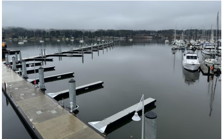
Construction of the new floating breakwater is complete!
