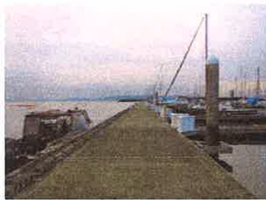
Example of a concrete pontoon floating breakwater.
