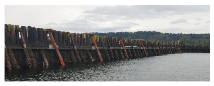
The existing breakwater is comprised of a vertical soldier pile wall. Numerous piles have failed and offer no structural integrity to the breakwater.
