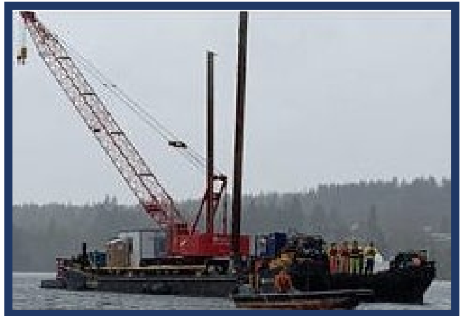
Marine borings were taken to evaluate geotechnical conditions for pile driving
